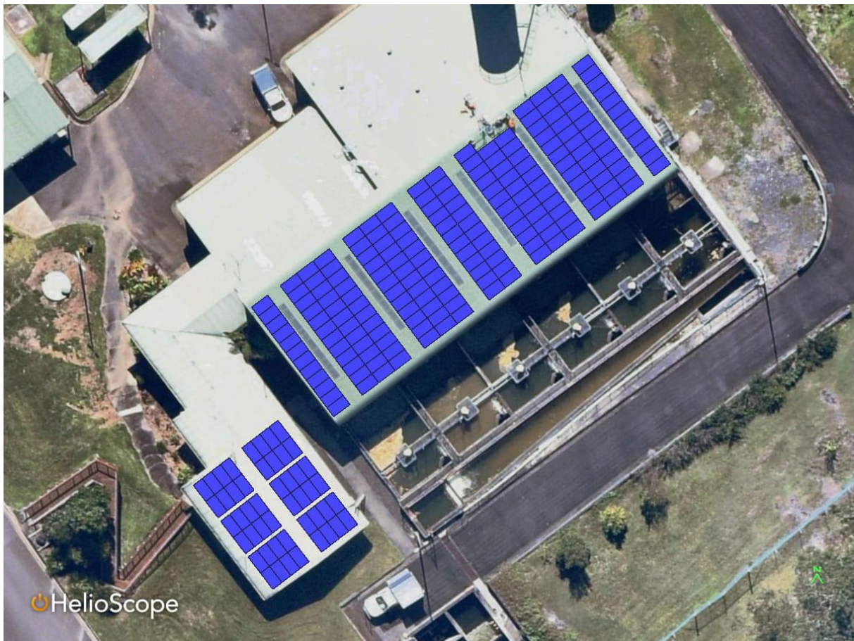
FIGURE 47: NIGHTCAP WATER TREATMENT PLANT ~100-KW SOLAR PV SYSTEM (RE-MODELLED)
